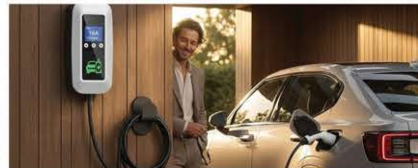
EV Car Charging Point
